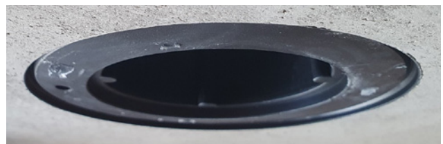
After pouring concrete, only a closing edge is visible. No post-treatment required.
